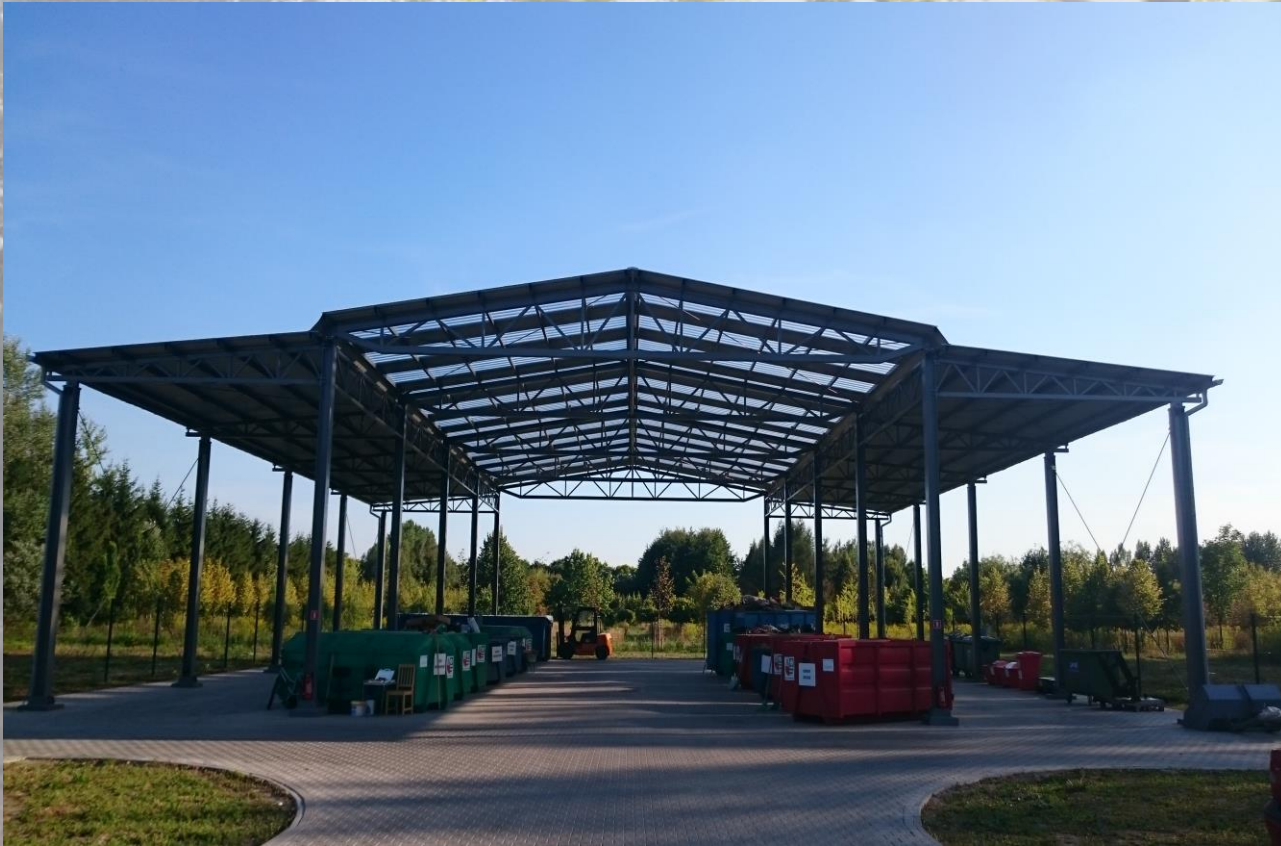
COMMUNAL WASTE COLLECTION POINT
